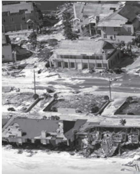
Devastation from Hurricane Ivan.
